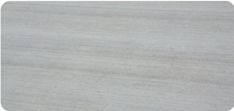
Broom brush concrete footpath
